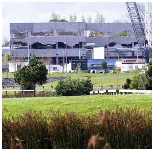
The Crossing under development at Highbrook Business Park, East Tamaki, Auckland.
