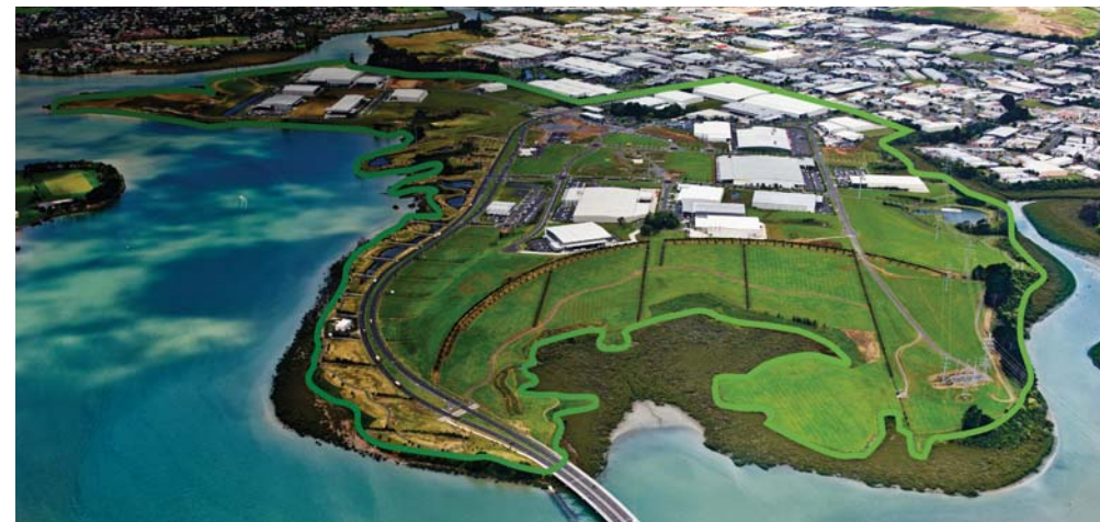
Aerial view of Highbrook Business Park, East Tamaki, Auckland.
