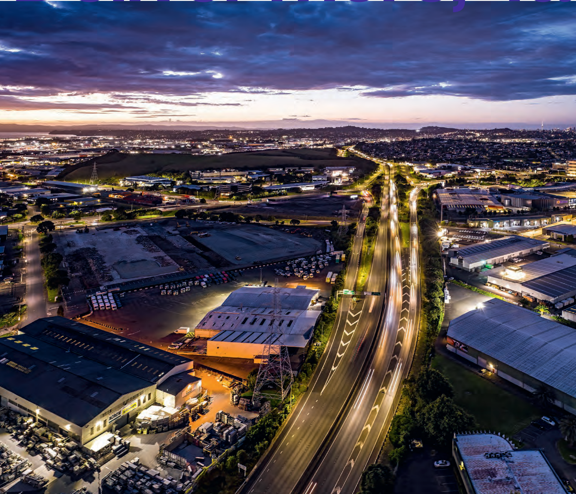
View over Mt Wellington Estate during earthworks March 2026.
