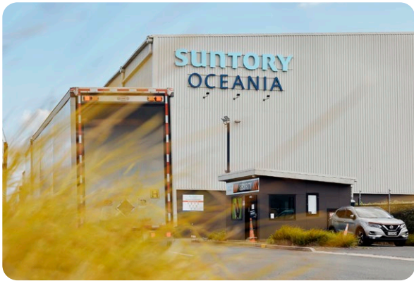
Suntory Oceania’s Auckland warehouse, ‘The Vault’, was purpose-built in 2013 and is located at Goodman NZ’s M20 Business Park in Manukau.
