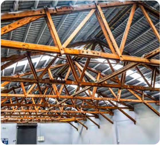
Stunning wooden rafters feature in Building 6
