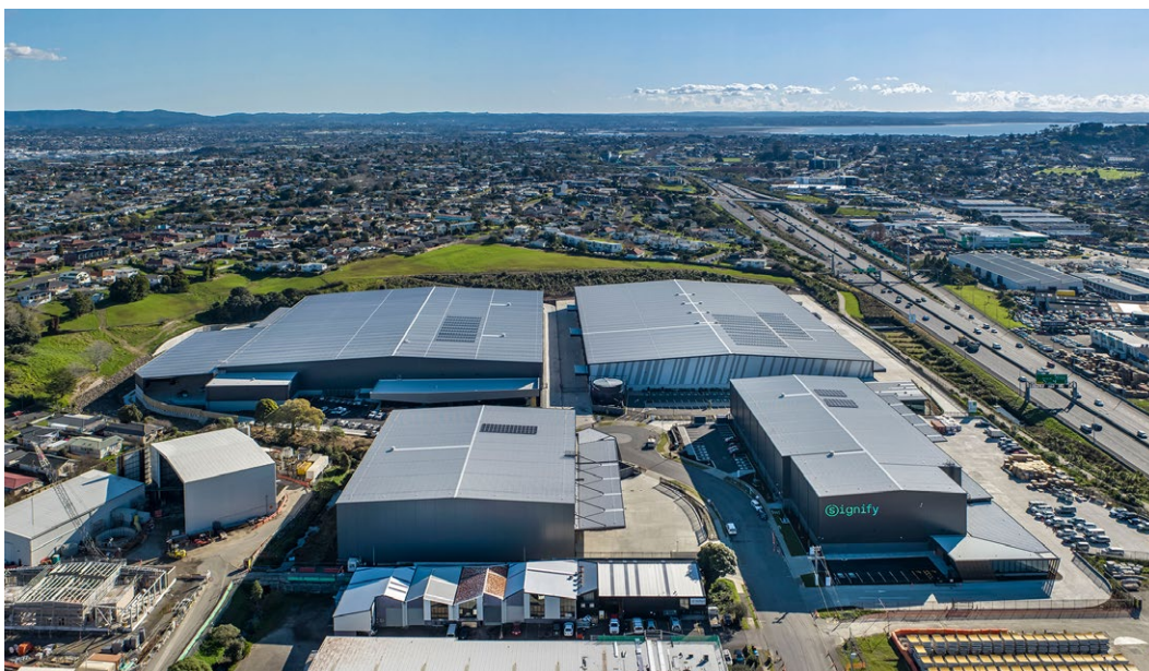
Roma Road Estate, Mt Roskill The redevelopment of Roma Road Estate is now complete. Cotton On, NZ Post and Signify are the customers that have chosen the central Auckland location alongside SH20.
