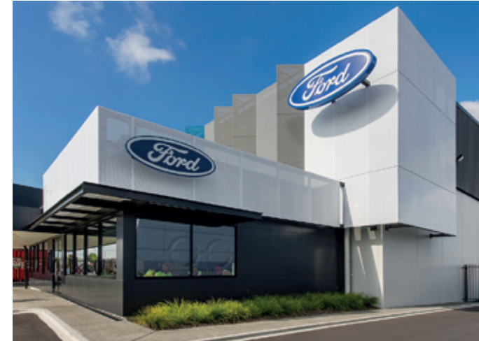
Highbrook Business Park Ford New Zealand Warehouse
