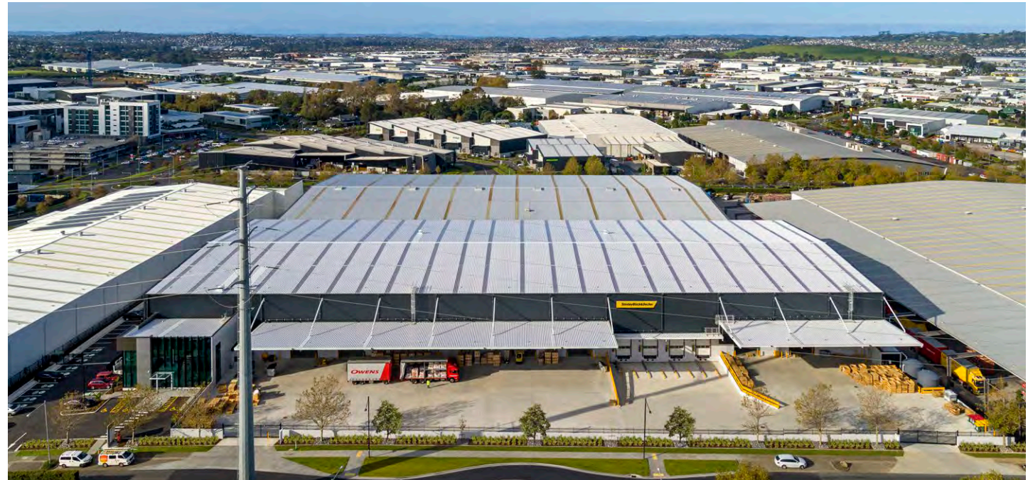
7 Stanley Black and Decker, one of the three development projects to complete at Highbrook Business Park in FY23.
