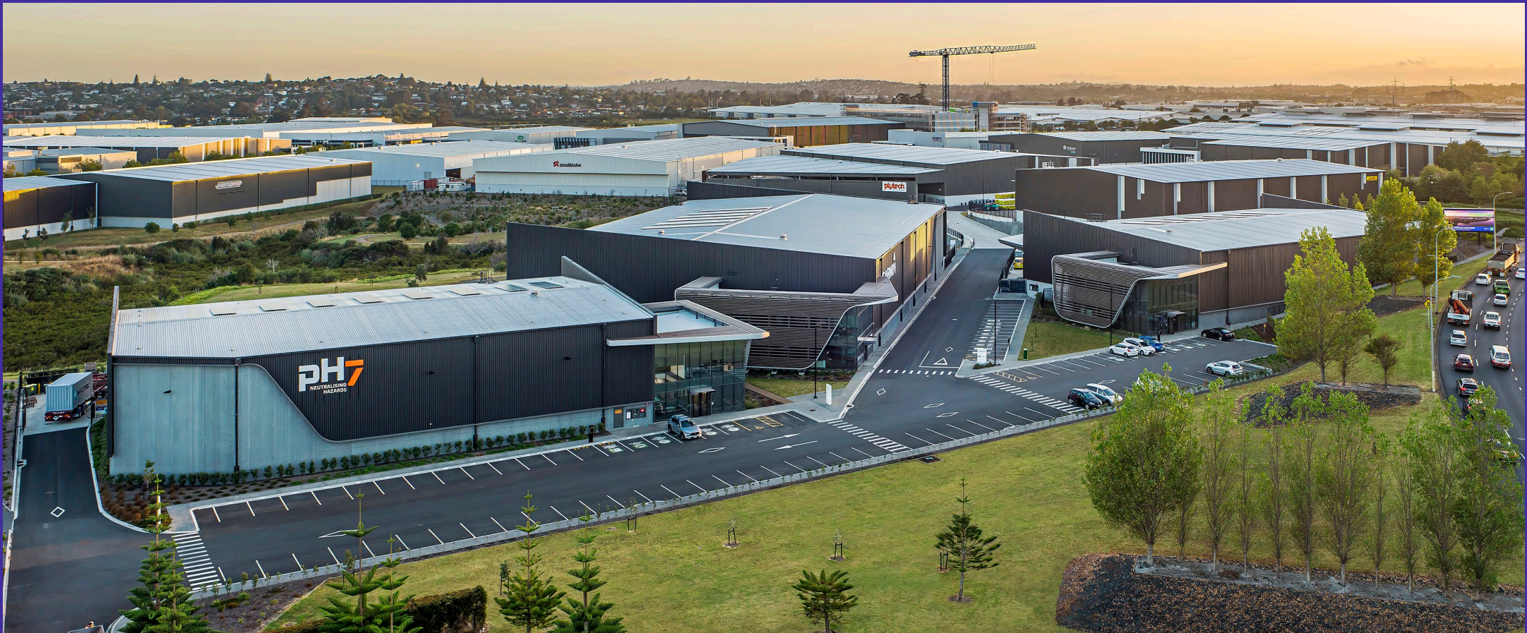
Three stand-alone buildings across 8,315 sqm, leased by pH7, Garmin and Chemist Warehouse.
